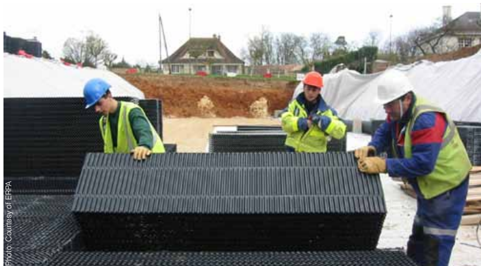
Ultra lightweight water-bearing modules made from recycled rigid PVC films
